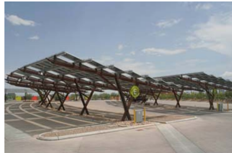
Figure 11: Springs Preserve Bifacial Fixed Installation
